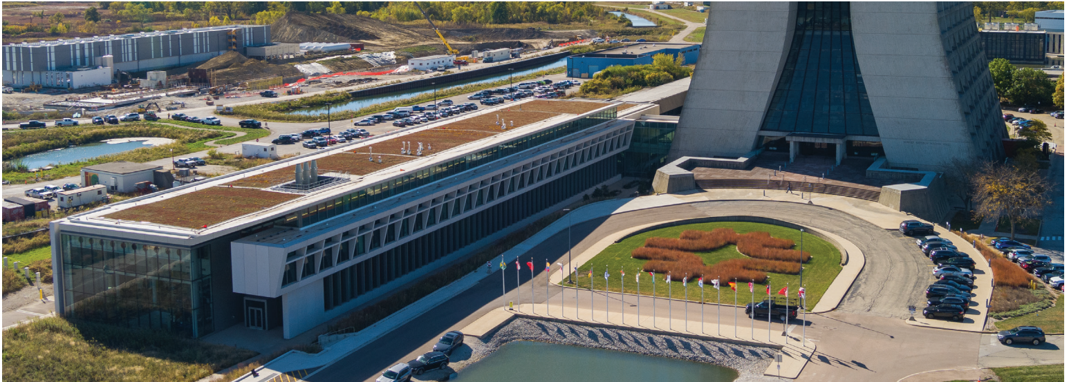
The Helen Edwards Engineering Research Center connects to the lab's 16-story office building, Wilson Hall. Photo: Ryan Postel, Fermilab
